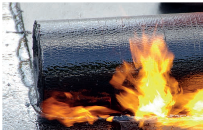
图3: 火焰加热Lucobridge®BIT
