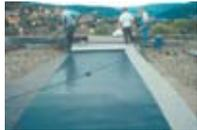
Laying and welding new roofing and sealing membranes
