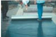
Protection layer on old bituminous sealing
