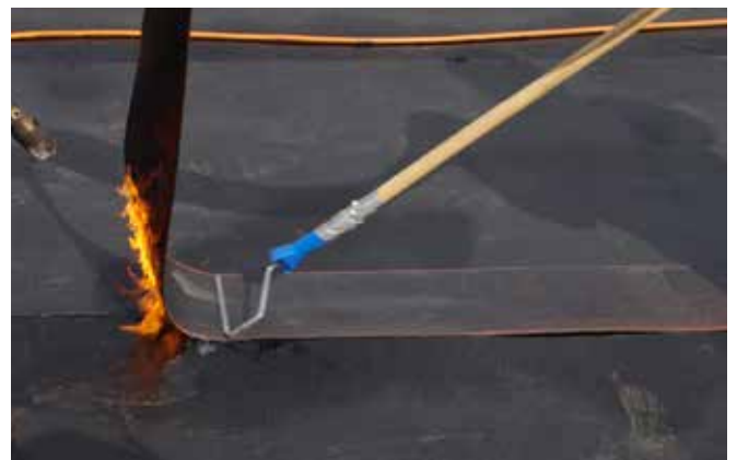
Figure 5: Laying edge-to-edge membranes
