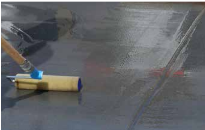
Figure 2: Priming the surface
