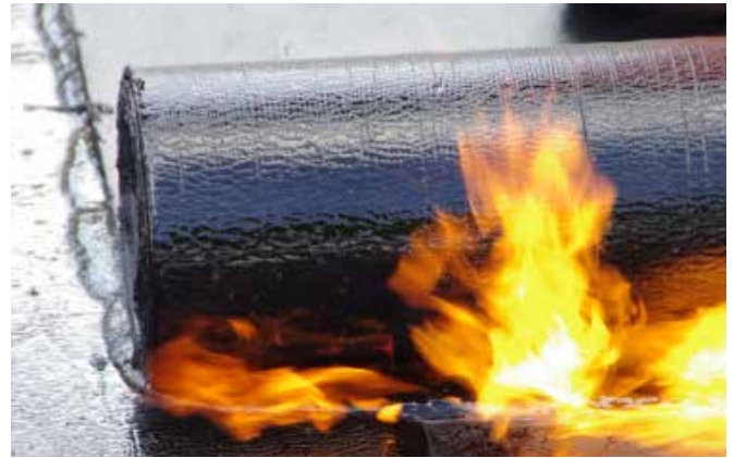
Figure 3: Flaming the membrane
