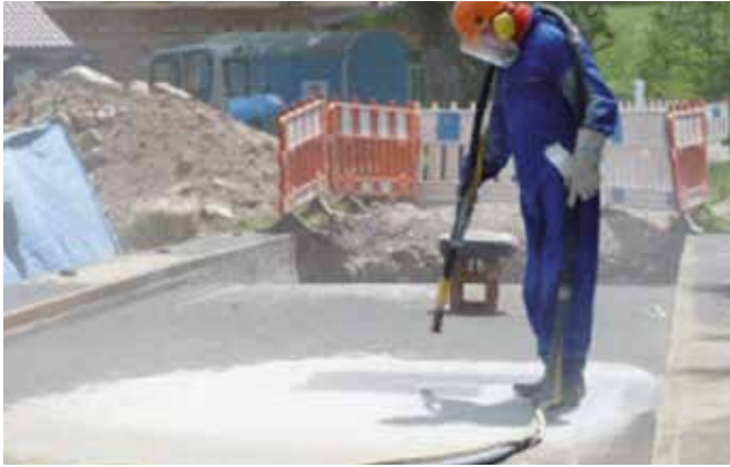
Figure 1: Remove the old surface
