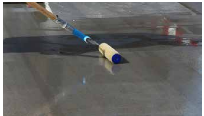
Figure 9: Priming the surface
