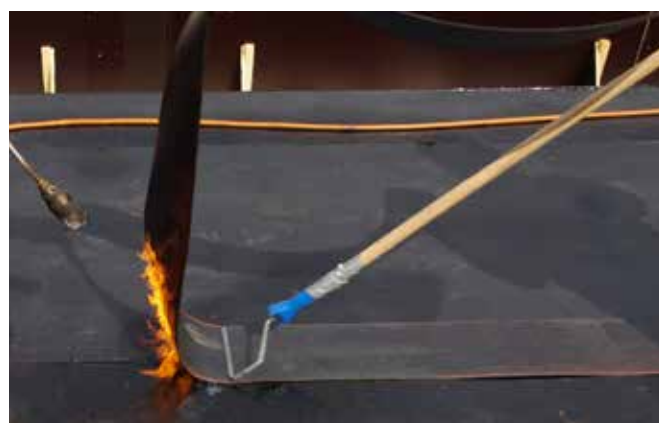
Figure 4: Laying edge-to-edge membranes
