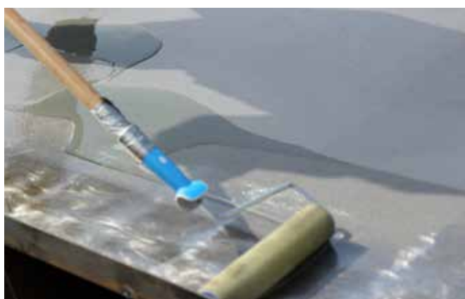
Figure 2: Priming the surface
