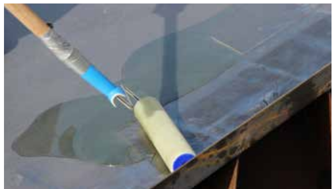
Figure 8: Priming the surface
