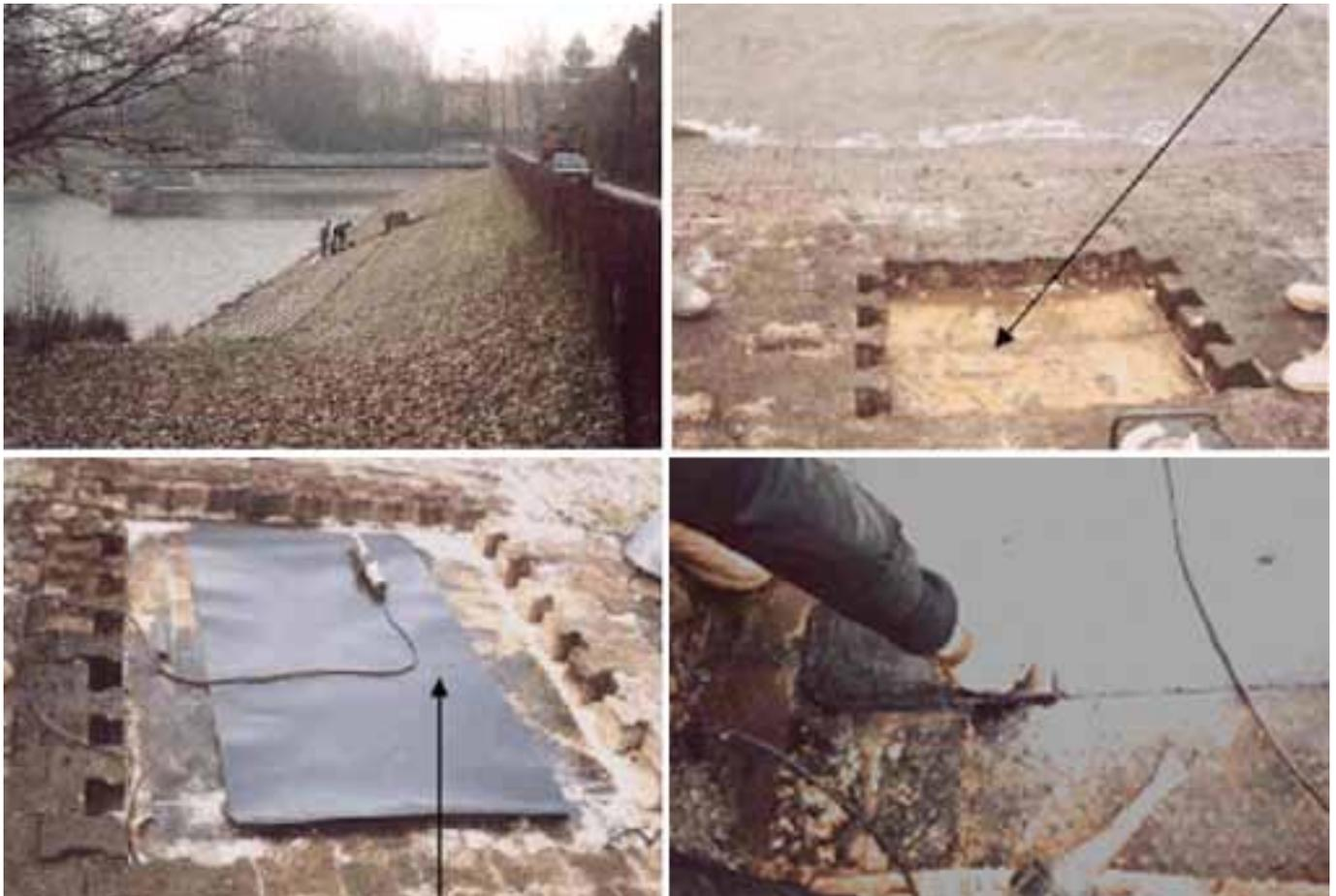
Image 14: Extraction of material sample from the sealing at the "Embankment Dam Kell" and subsequent closing of the hole by means of hot gas welding, 2004.
