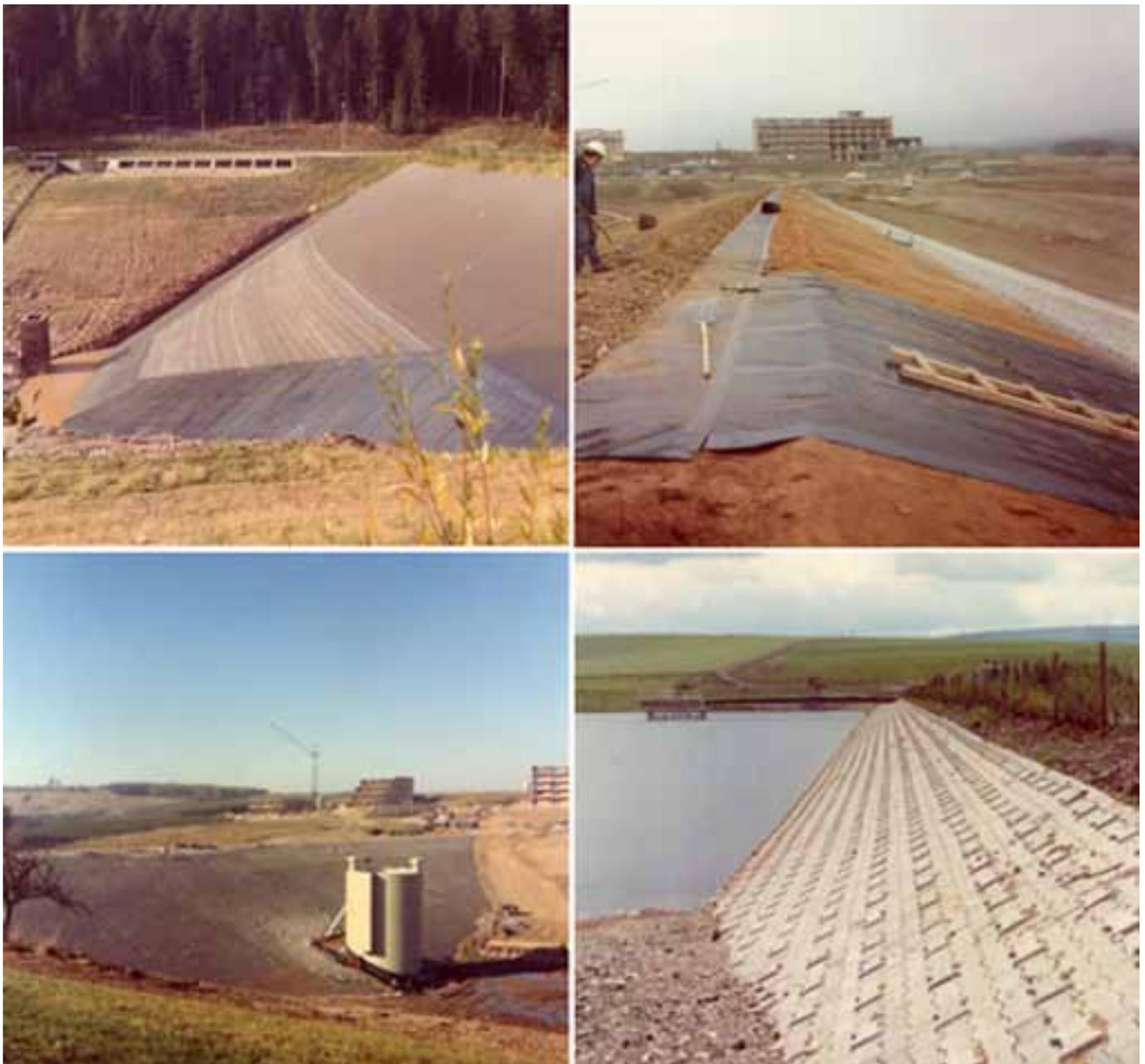
Image 13: Sealing of embankment dam at "Keller Stausee" with sealing sheets made from Lucobit 1210, 1971
