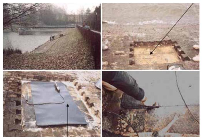
Image 14: Extraction of material sample from the sealing at the "Embankment Dam Kell" and subsequent closing of the hole by means of hot gas welding, 2004.
